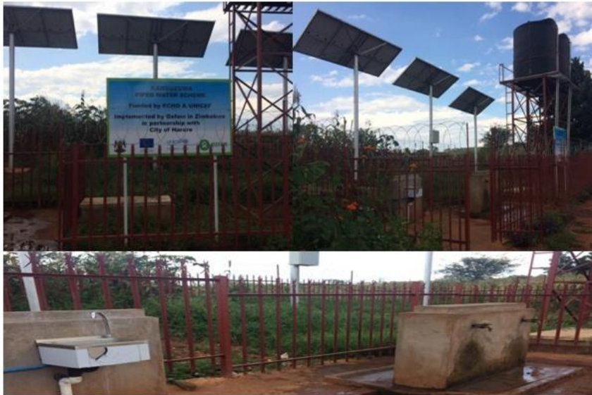
Figure 2: An upgrade of the Kambuzuma section 1 borehole (Authors, 2021).
